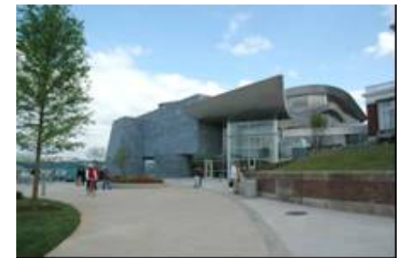
Museum of American Art, Chatanooga (USA) Architect: Randall Stout Architects CDROM ref: PX SPEC – PX AUDACE
