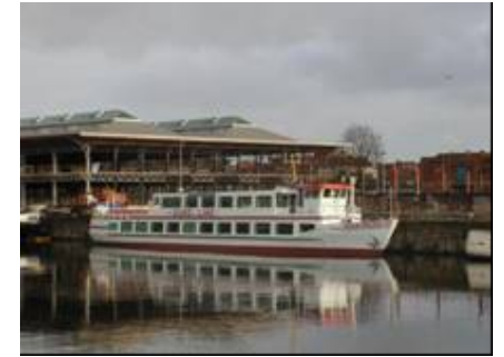
Renovation of a warehouse in a Shopping Centre, Ghent (Belgium) Architect: Romain Berteloot CDROM ref: PX SPEC – PX TRAD
