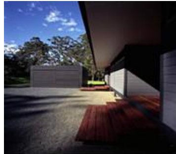
House in Foxgraound (Australia) Architect: Rita Qasabian CDROM ref: HAB IND – ME AUS
