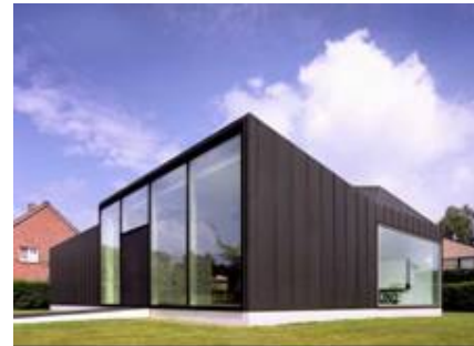
Offices in Ghent (Belgium) Architects: Arlauskas Arunas & Eckels Armand CDROM ref: PX SPEC – PX JURY
