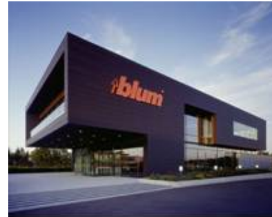
Offices and showroom, Herford (Germany) Architect: Dirk Stanczus CDROM ref: LI ENTR – ME IT
